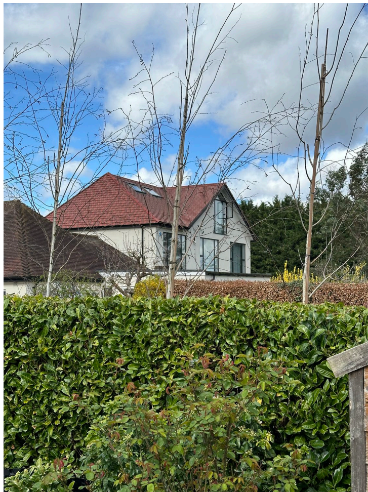
Figure 22 – Photo of Hillyfields (No.11 Hayes Mead Road)
